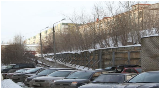
Fig.1. Retaining wall with retaining constructions
