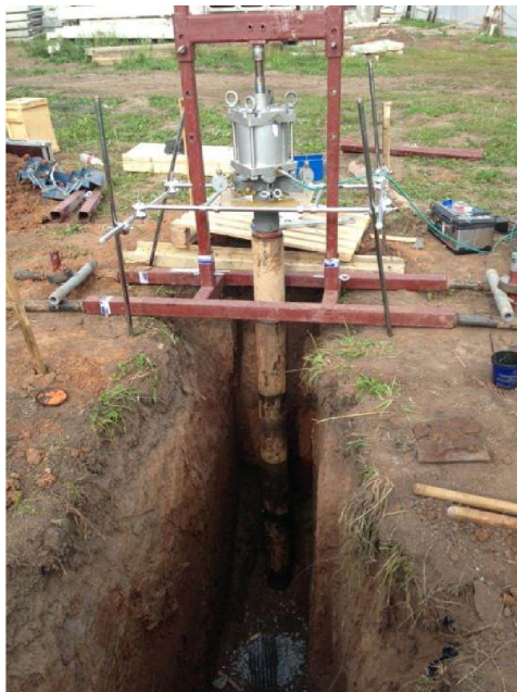
Figure 2. General view of the pit for testing
