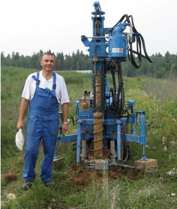
Figure 2. Borehole drilling on the top of MSW mass.
